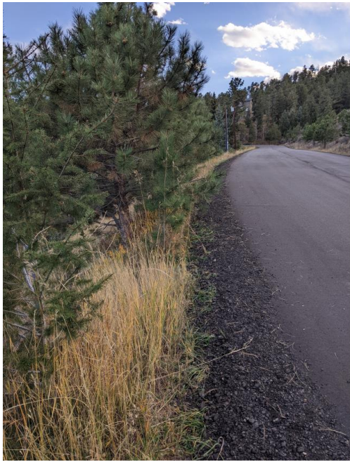
Figure 4.1-1 Trees Overhanging the Road.
